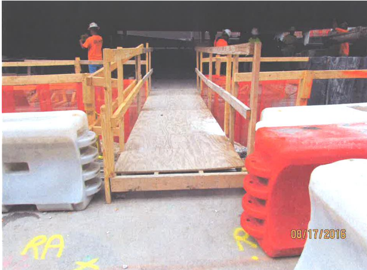
Photo 2 of 2 – The wooden bridge built for employees to enter the parking garage located approximately 60 feet for the area where the incident occurred.
