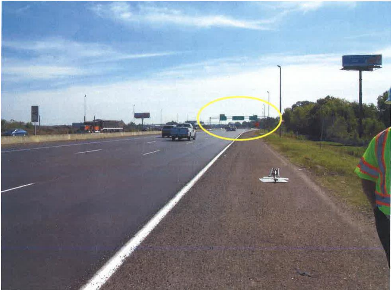
Photo 1 of 1: Eastbound lanes of I40 near the Exit 12A, the yellow oval designates the approximate area where the incident occurred.
