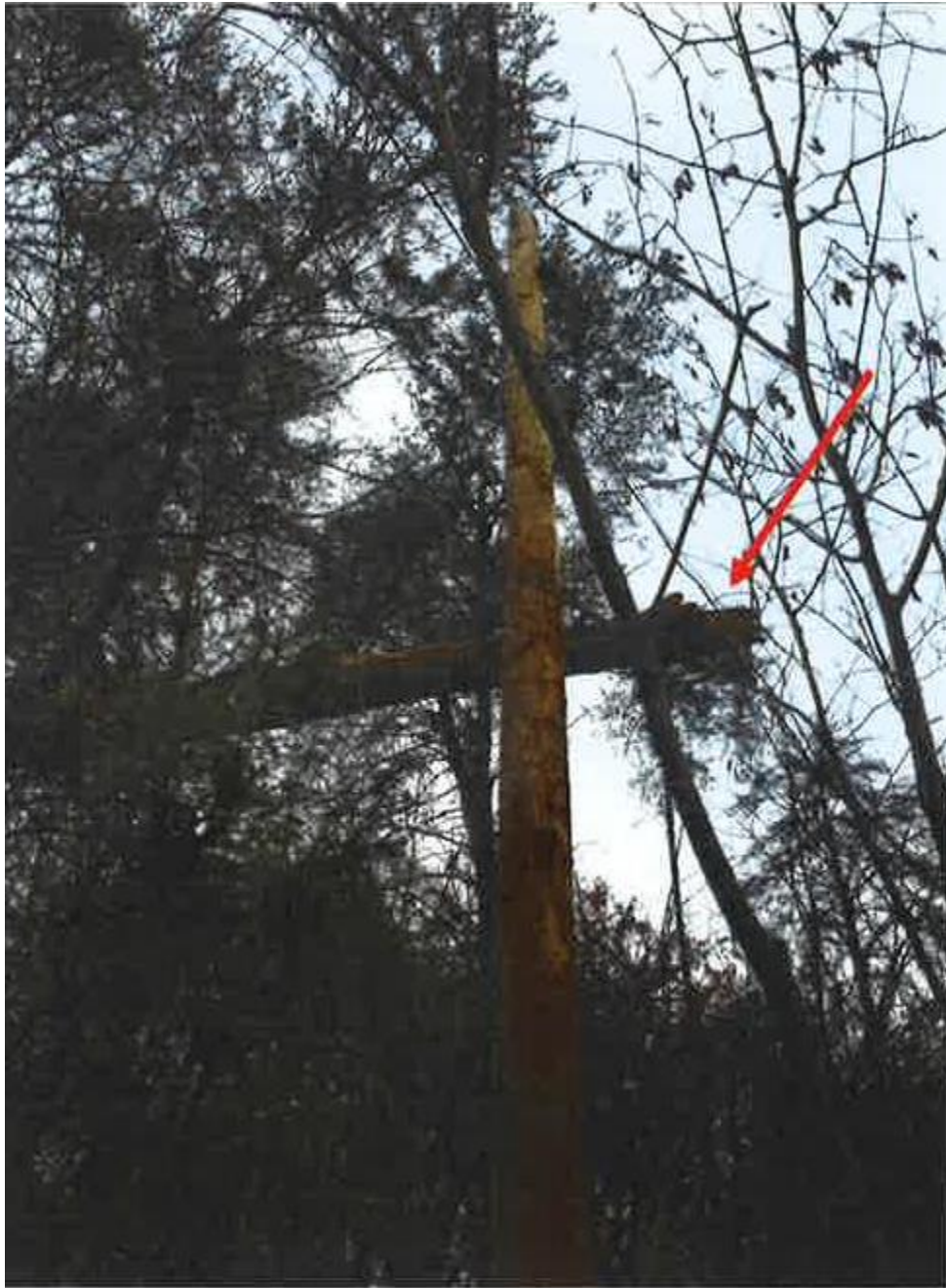
Photo 1 of 1 – Rotten tree hanging on cable lines as indicated by red arrow.
