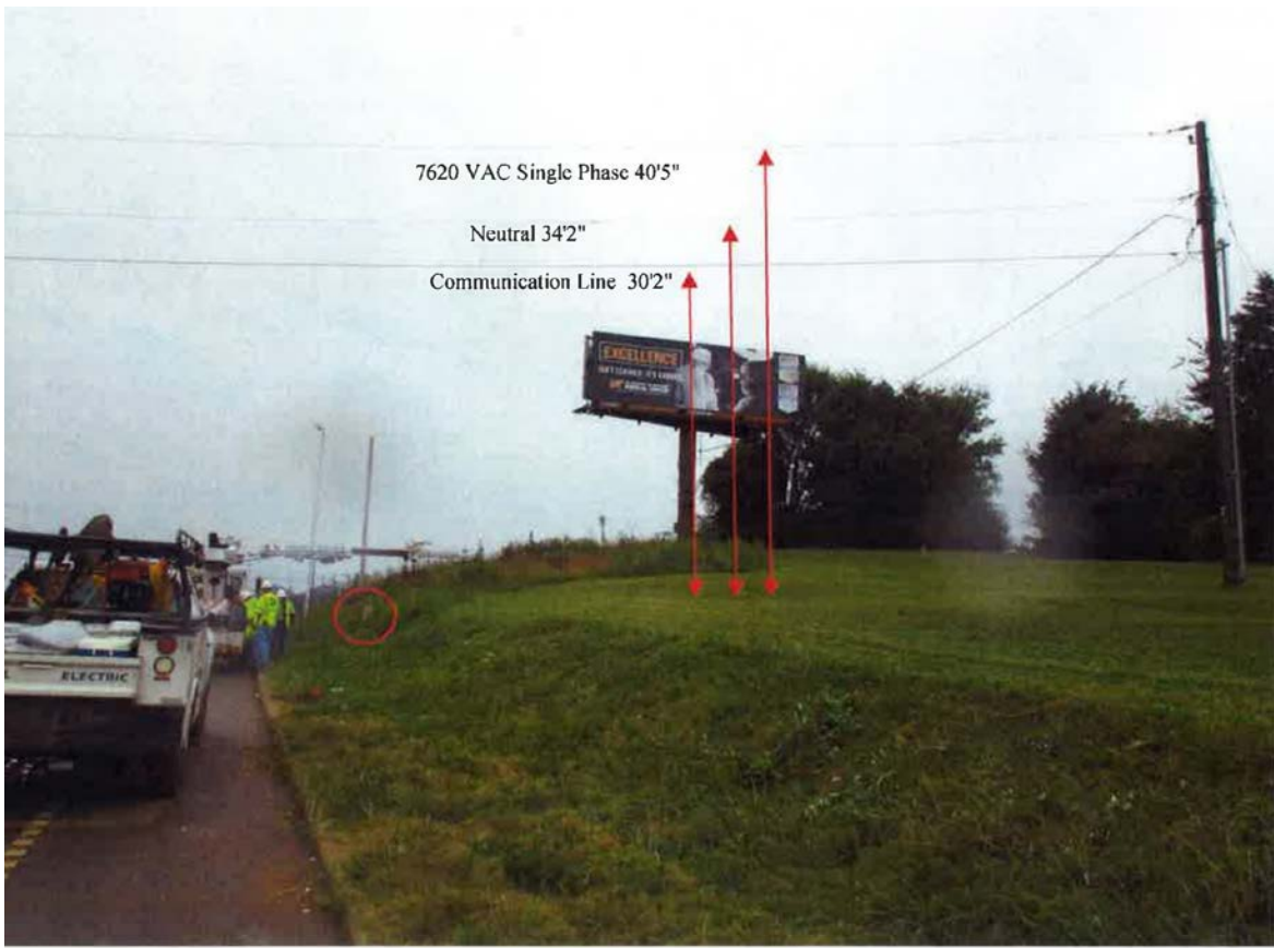
Photo 1 of 1 – Photo shows an overall view of the incident scene. The overhead powerlines are identified with the red arrows. The red circle indicates the original location of the street light pole.
