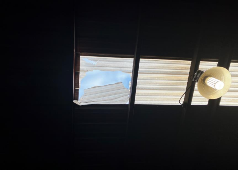
10 Fall through skylight—Insp #1721951 Big G Metal Works Inc.
